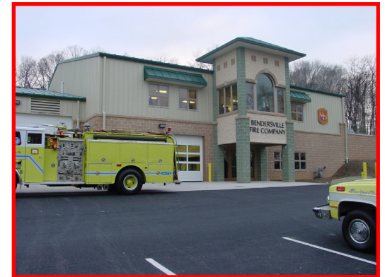
In 2002, the first loan was granted, providing Bendersville Fire Company in Adams County with $125,000 to assist with construction of a new community building and fire station.
